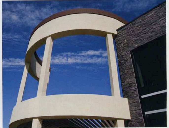
Inviting architectural accents and exterior waterscapes bring a sense of tranquility before you enter the reception lounge.
